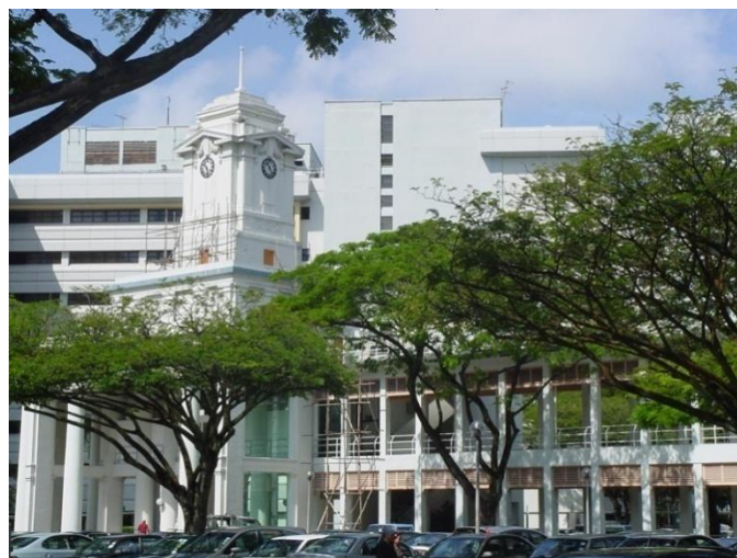
Clock Tower and part of the walkway comprising the Bowyer Block
